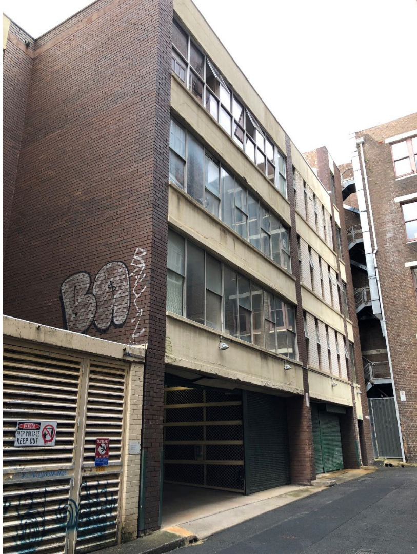
site viewed from St Barnabas Street looking west
